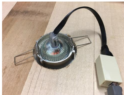
View from above the ceiling
