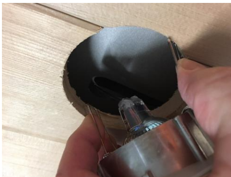
Compress retainers and insert into hole
